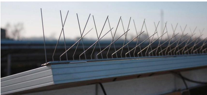
Figure 8: Metal spikes on PV modules to deter birds [17]
