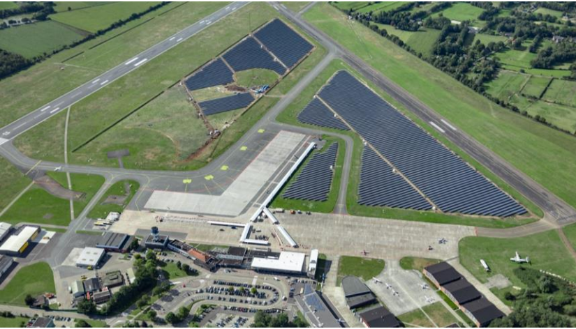
Figure 3: Netherlands - Groningen Airport, 21.9 MW installed capacity, between runway and taxiway [5]
