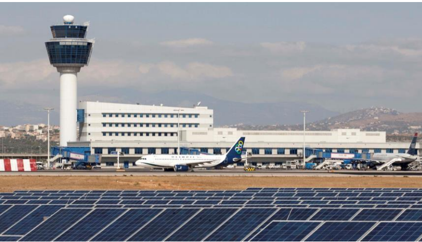
Figure 4: Greece - Athens International Airport, 16 MW installed capacity next to runway [6]
