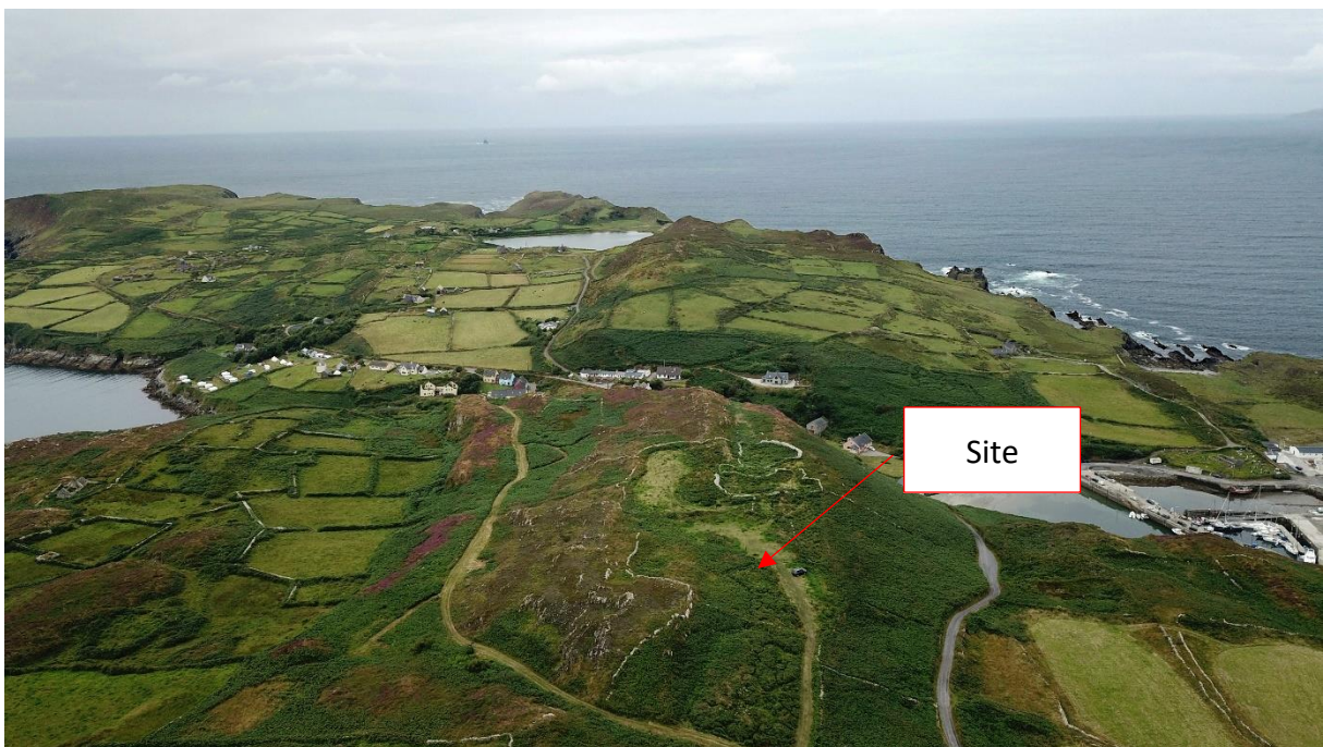
Figure 6: Drone image of the site (2/2). Courtesy of Ciaran O Driscoll.
