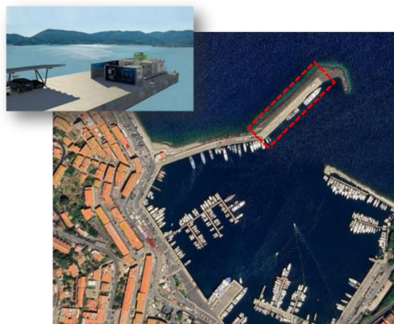
Figure 22: view of the Porto S. Stefano identified deck area in the port and a rendering of a hydrogen refuelling station on a pier (credits Bzero)
