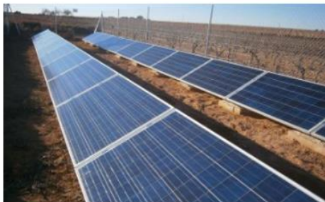
Figure 6 - Flat surface concrete mounting system.
