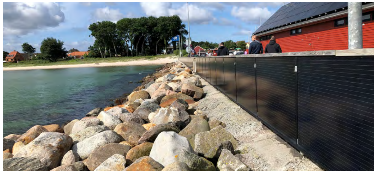
↑ The marina on Samsø has been upgraded with a solar PV and battery installation allowing the harbour to produce its own renewable electricity. © Photo by Marina Montero Carrero
