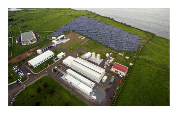
A megawatt-scale grid-forming renewable energy system which combines wind power, solar power and a battery grid storage system, through an all-new energy infrastructure with 5,5 MW.
