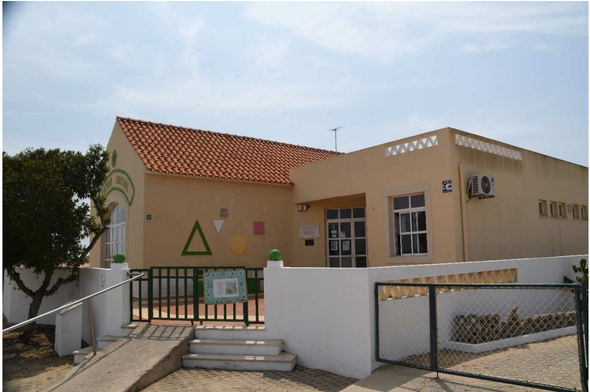
Figure 10: Central and south sector - kindergarten
