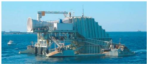
Figure 39: The sea bed mounted, fixed-structure OWC project in Port Kembla, Australia [28].
