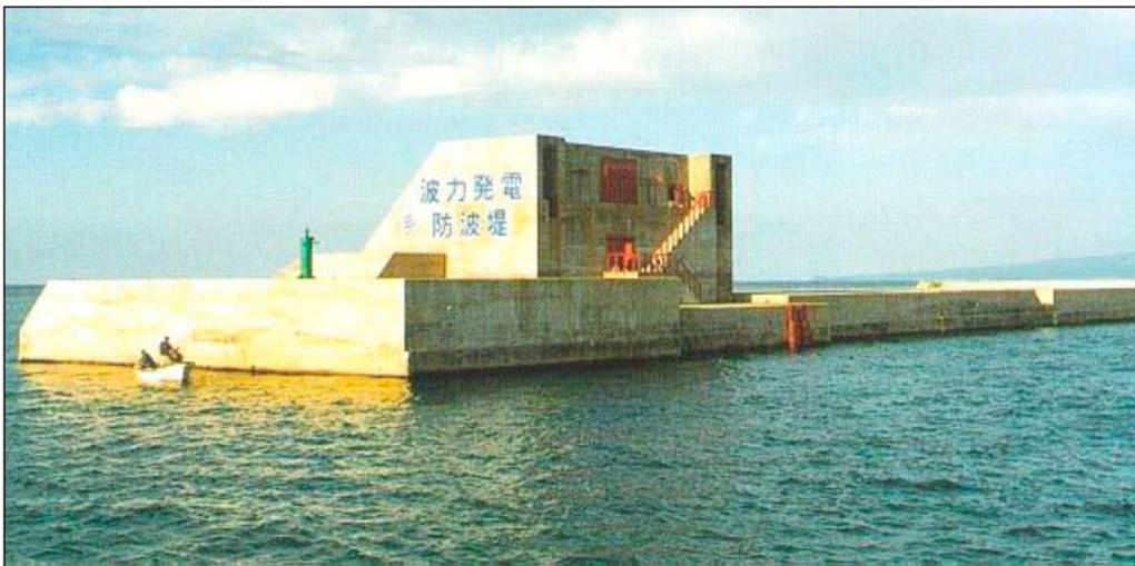
**Figure 40:** The fixed-structure OWC project in Sakata, Japan, mounted on the breakwater [28].
